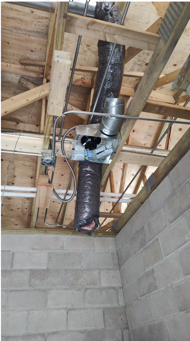
Photo 3: View duct and venting in place for exhaust, also can see the block chase wall complete.
