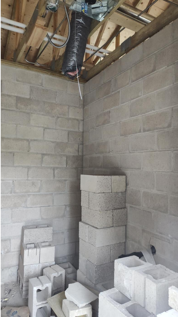
Photo 4: Block chase wall complete.
