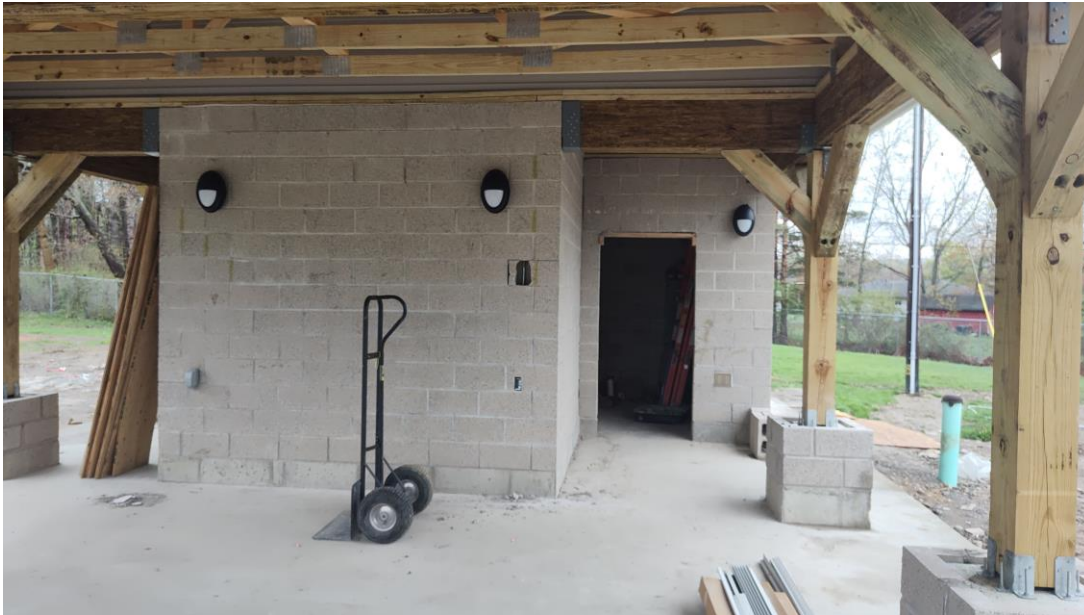
Photo 2: Exterior lighting installation.
