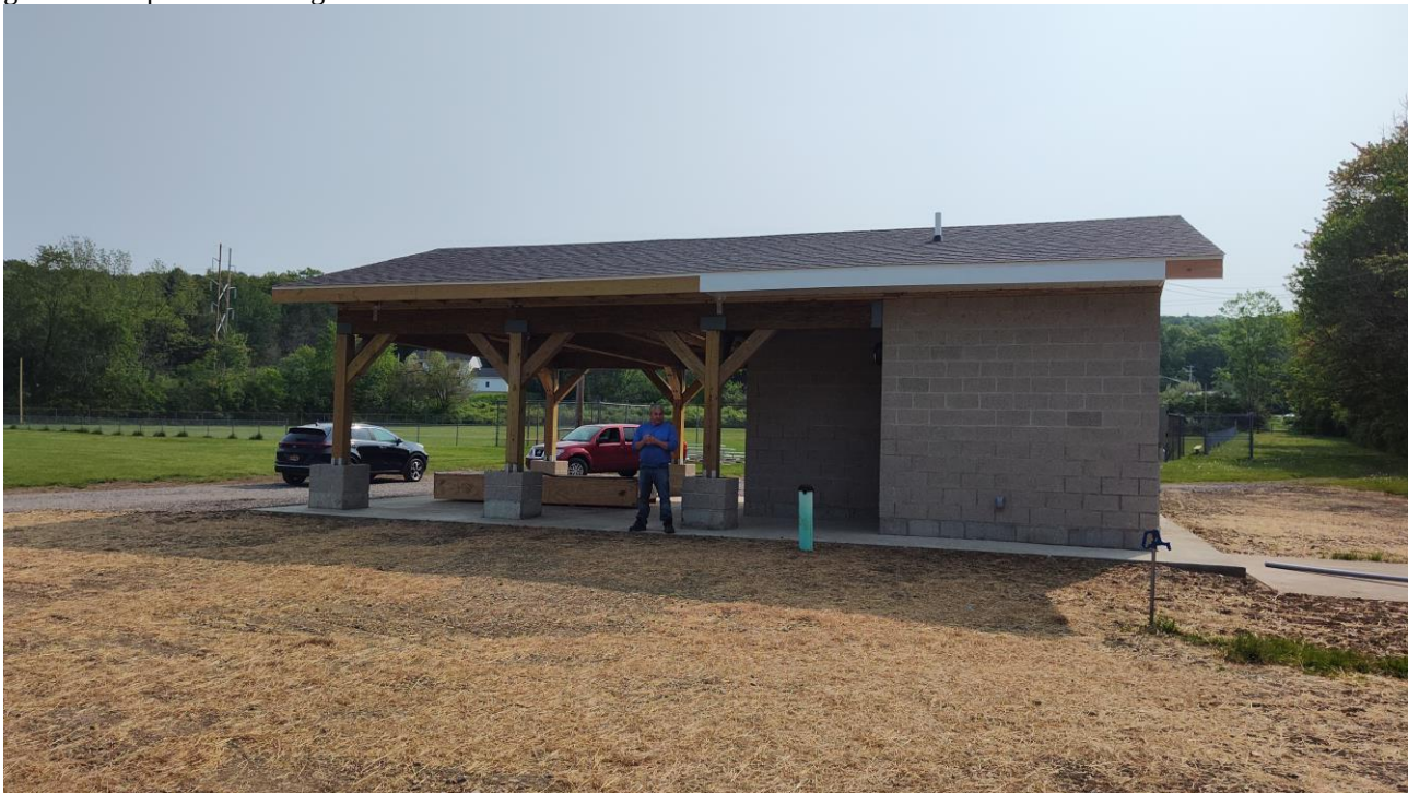
Photo 3: View of work in progress at pavilion. Sitework restoration in progress.
