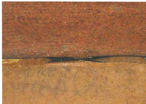
54. Voids in material along shell-to-floor connection.
