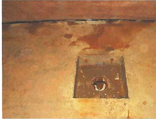
58. Corrosion on piping in sump.
