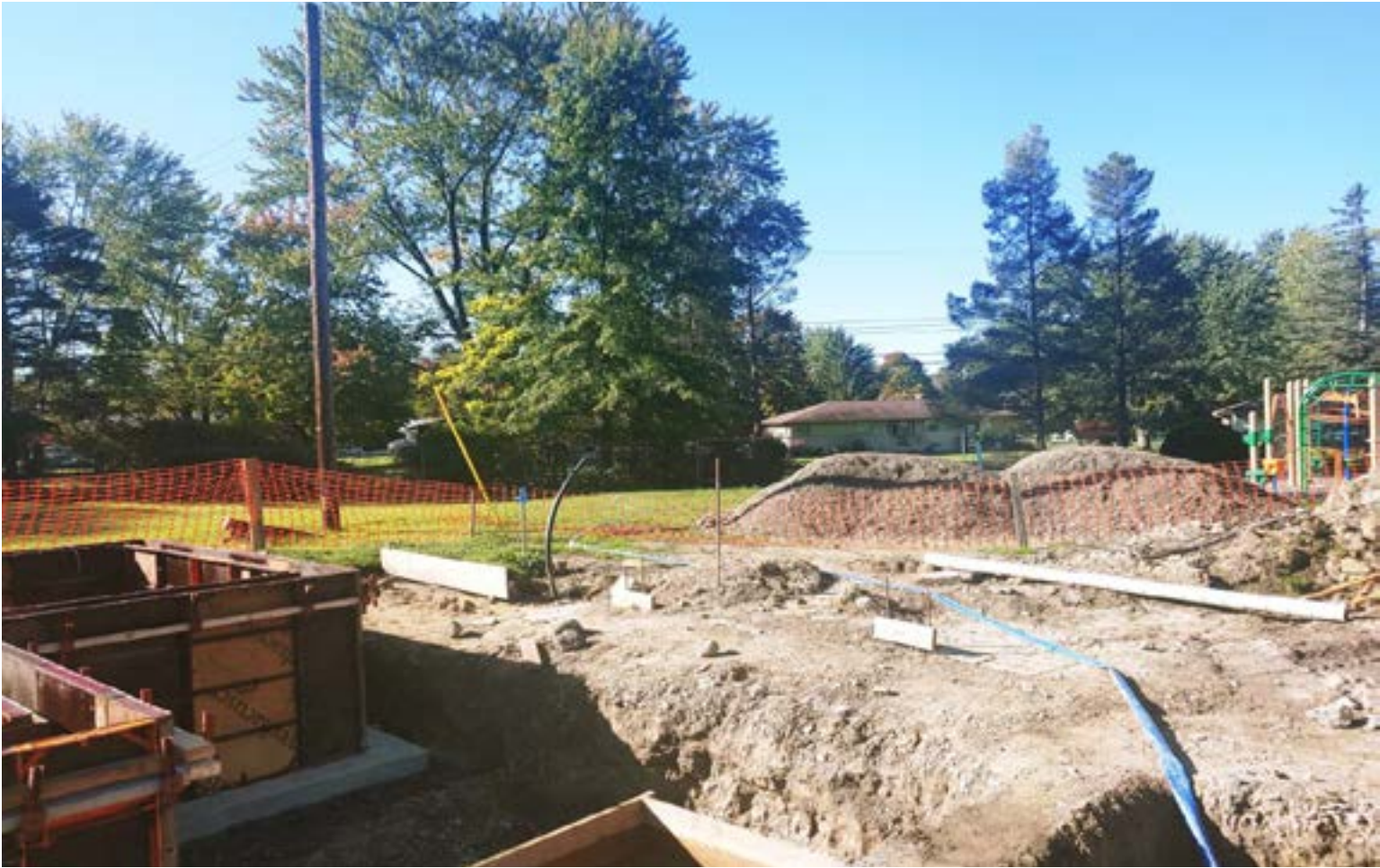
Image 2.7: Boston Drainage Project, 2021
