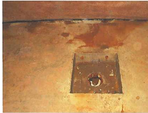
58. Corrosion on piping in sump.
