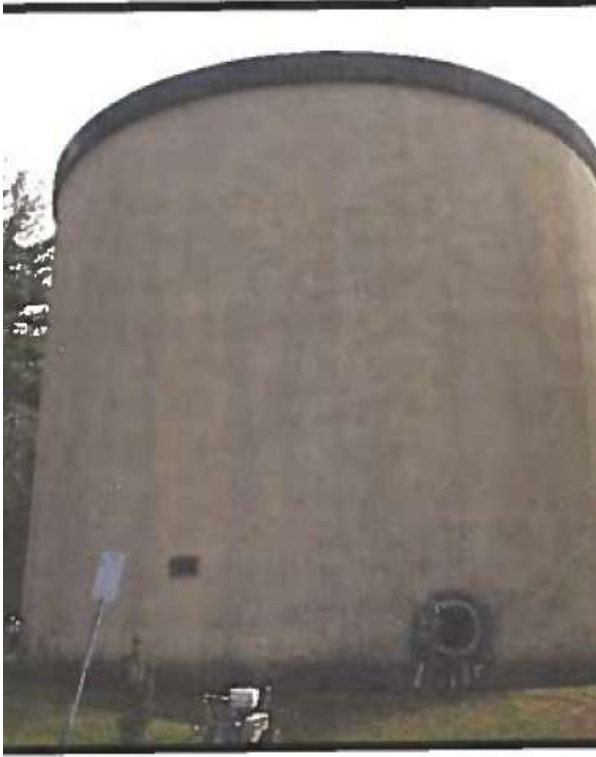
Water District 1 – Crestwood Tank
