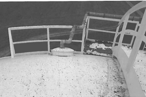
Roof safety railing, platform, stairs, and pipe attached to hinged roof manhole cover.
