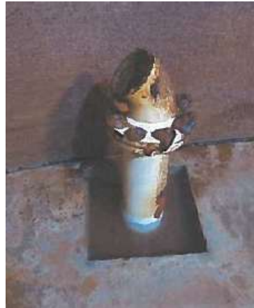
58. Corrosion on piping in sump.
