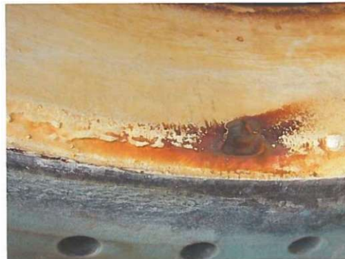
15. Corrosion and metal loss in shell manhole neck.
