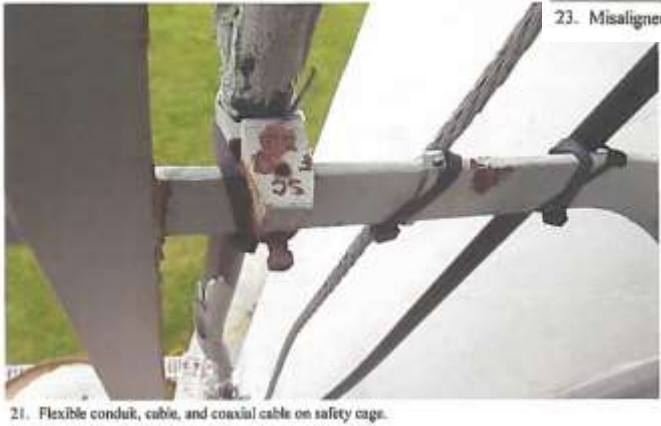
21. Flexible conduit, cable, and coaxial cable on safety cage.
