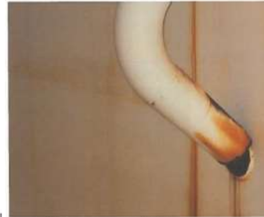
44. Overflow pipe no longer attached to shell.
