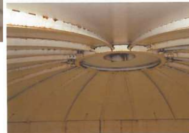
38. Corrosion on roof stiffeners.
