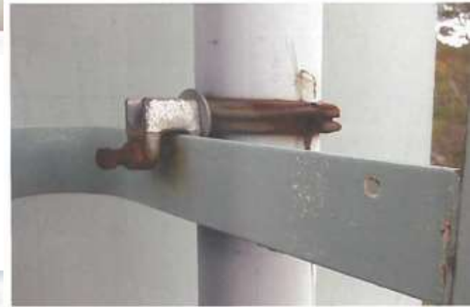
22. PVC pipe bolted to ladder safety cage.
