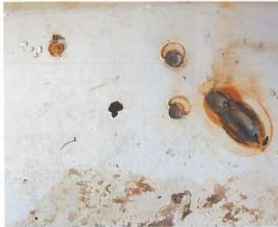
52. Metal loss in floor.
