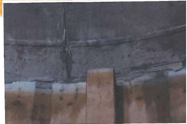
43. Concrete encasing overflow inlet.
