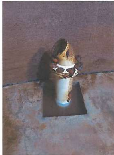
58. Corrosion on piping in sump.
