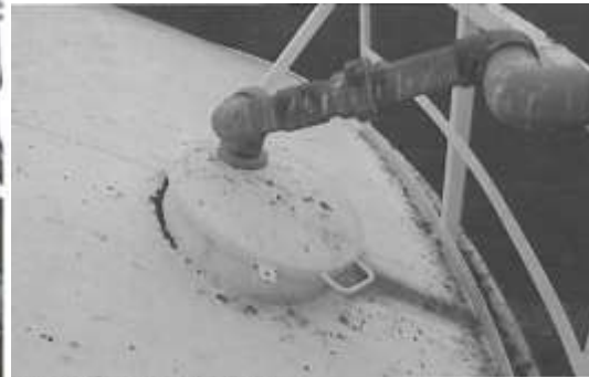
1. Pipe attached to hinged roof manhole cover.
