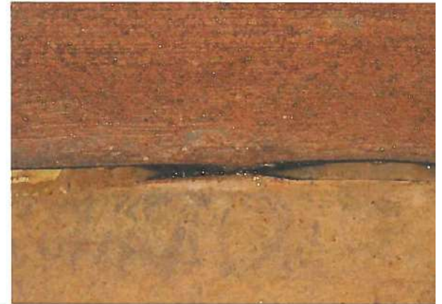
54. Voids in material along shell-to-floor connection.
