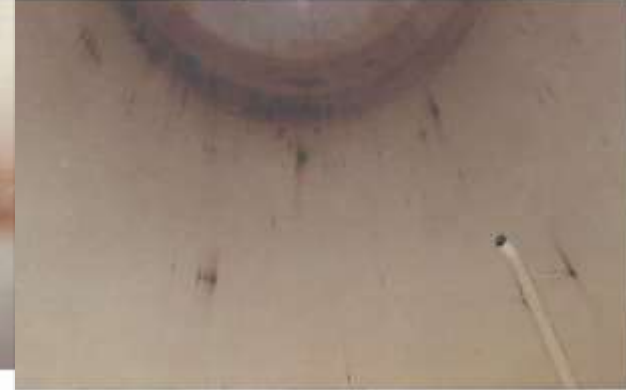
56. Corrosion on interior shell.
