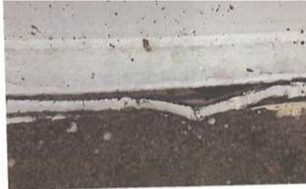
14. Peeled sealant along grout and bottom plate.
