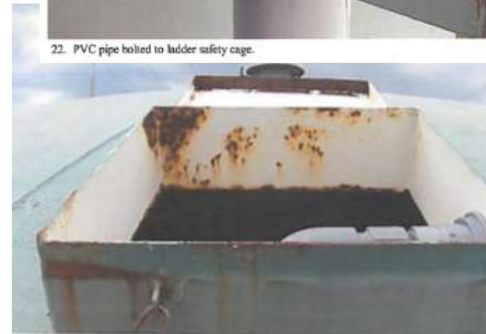
28. Corrosion on roof manhole.
