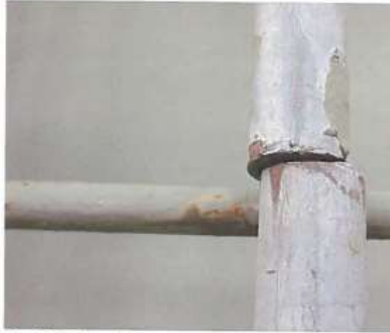
23. Misaligned notched-tubular rail sections.
