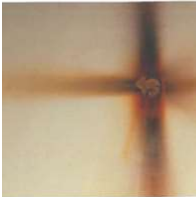
Corrosion on interior shell.
