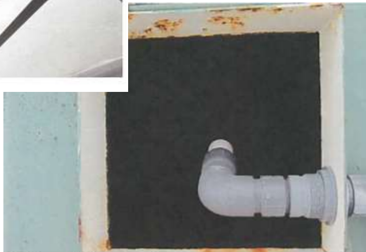
29. Piping extending into roof manhole.
