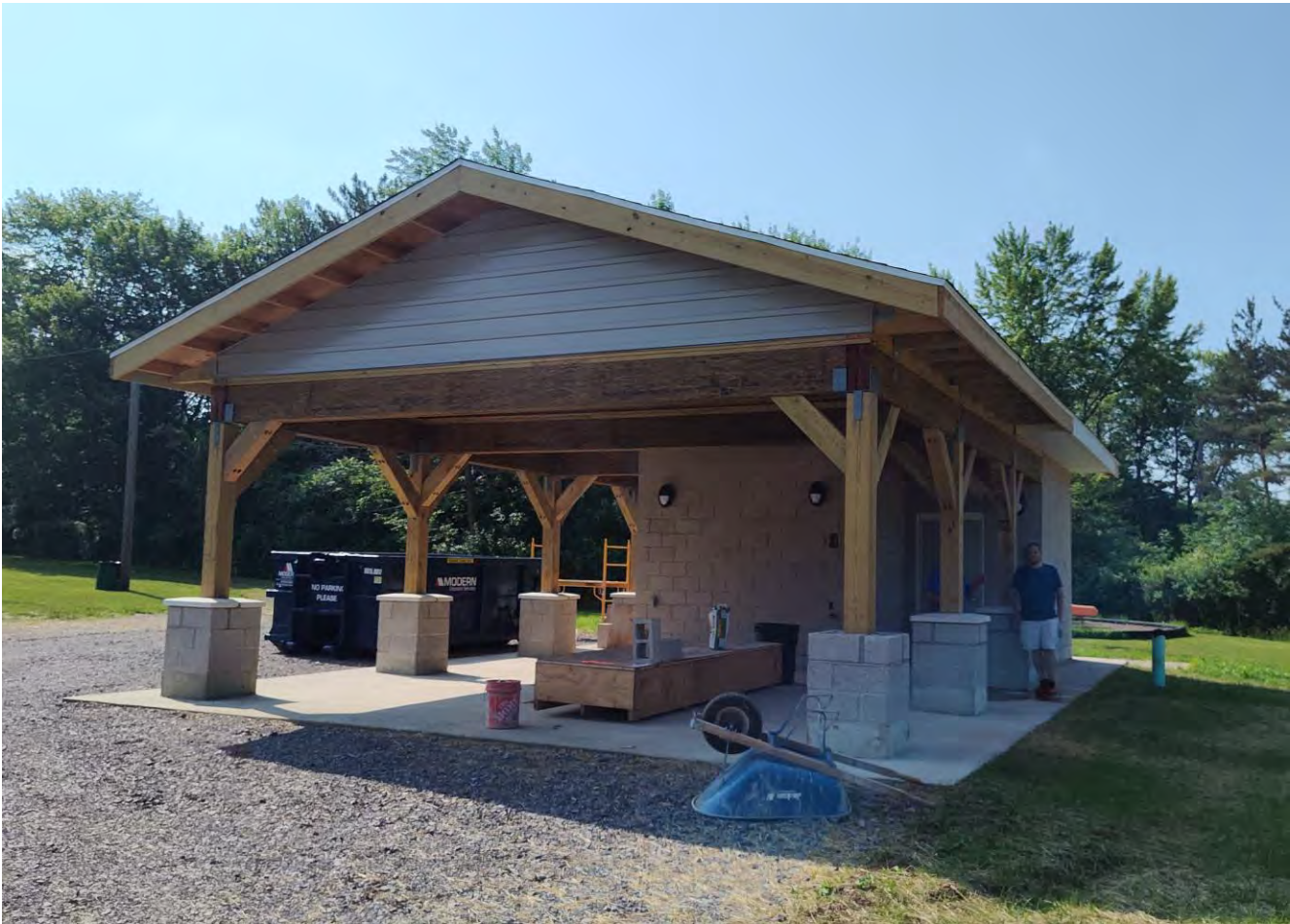
Photo 1: Photo of current site condition. As viewed the cap on the right front pier has not been installed.
