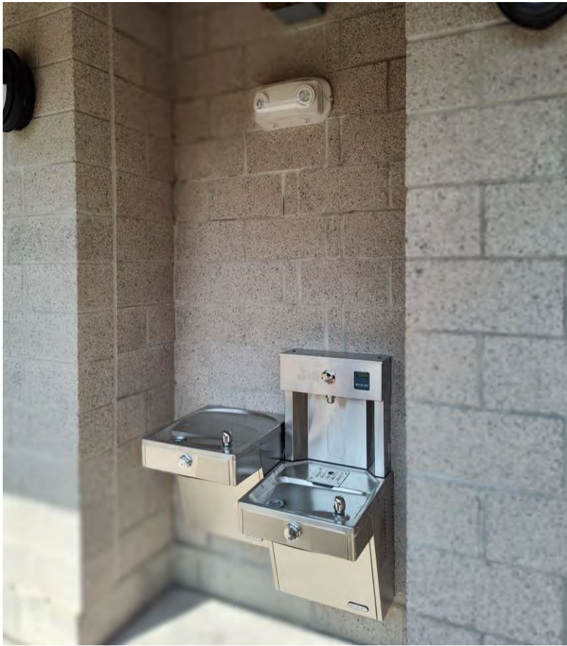
Photo 8: Drinking fountain/bottle filler installation, the bottle filler was not working – contractor to check with plumbing contractor to get it working.
