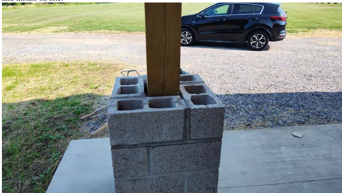
Photo 3: View of precast cap installation in progress- the last pier to receive a cap and be finished.
