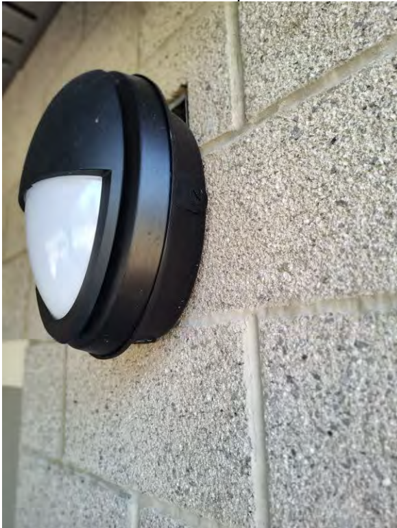
Photo 5: Block that needs to be repaired/ replaced at top of light fixture.
