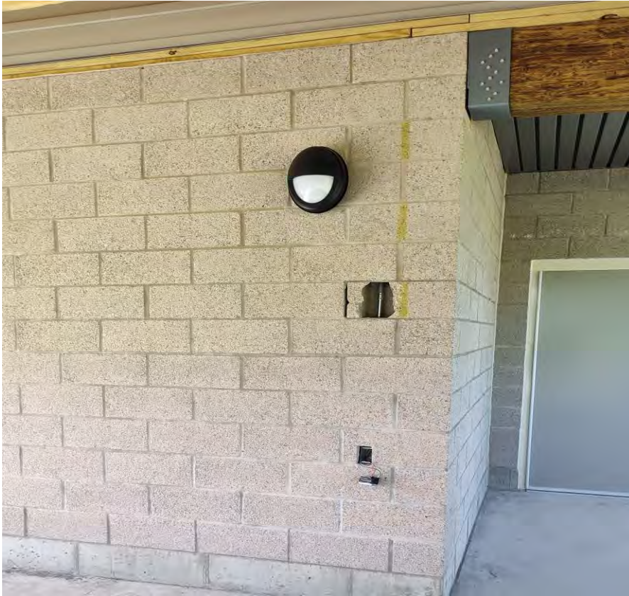
Photo 4: View of block to be replaced.
